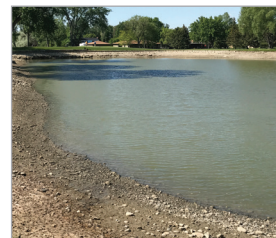
Irrigation pond used for roadside irrigation system.
